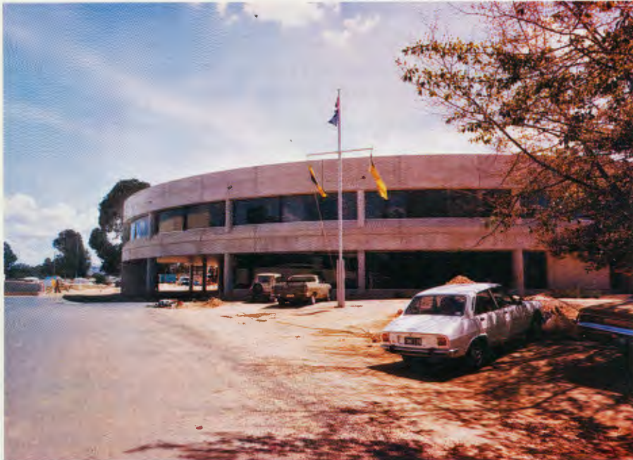
The Central Administration Building
